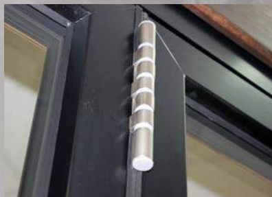
High security hinges, non face fixed.
